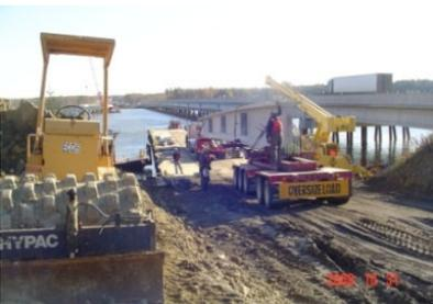
Beams were loaded onto barges and then erected by a barge-mounted crane.
