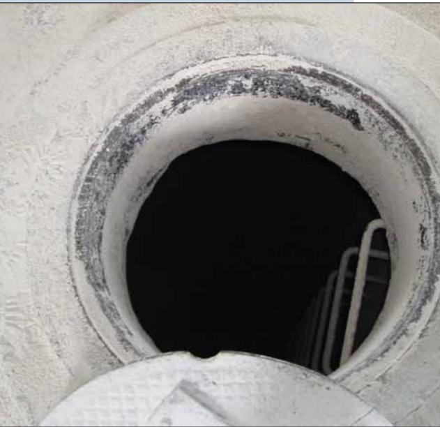
Simply taking the lid off of the lime bulk storage tank caused injuries to operators at a sanitary district in Mineral Ridge, Ohio.
