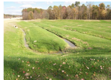
East Spill Containment Basin.
